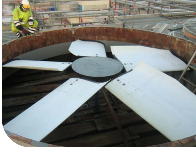
The new fan blades enabled a lower rotating speed, resulting in lower noise levels and reduced power consumption.
